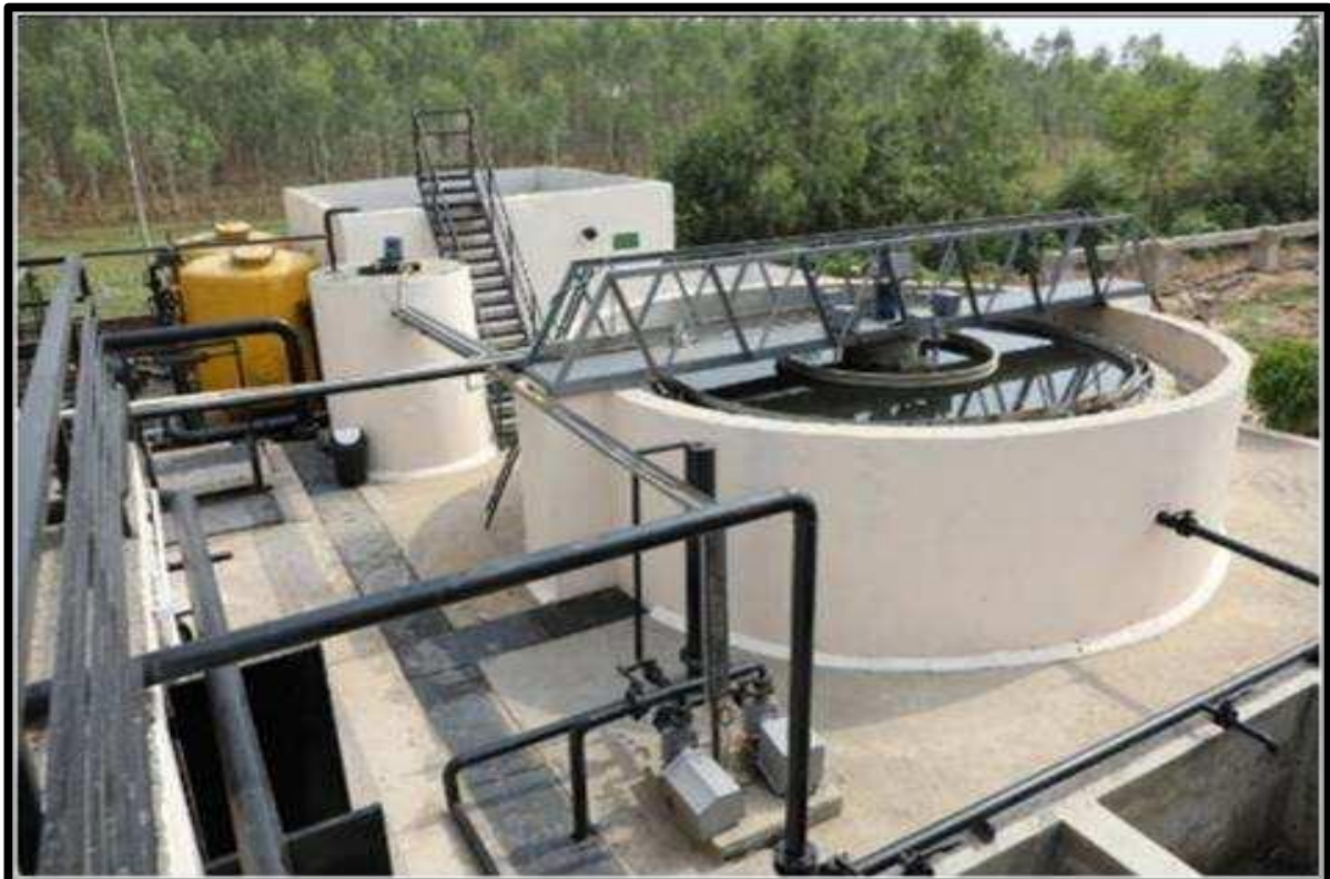
Treated wastewater being used in the campus and Sewage Treatment Plant of capacity 1 MLD
