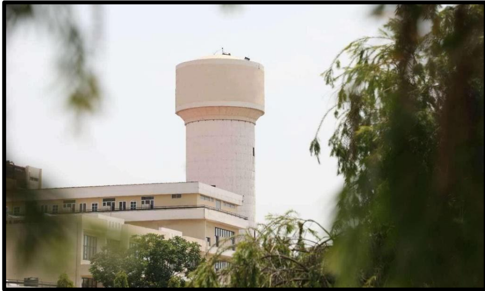
Overhead Tank of Capacity 400KL
