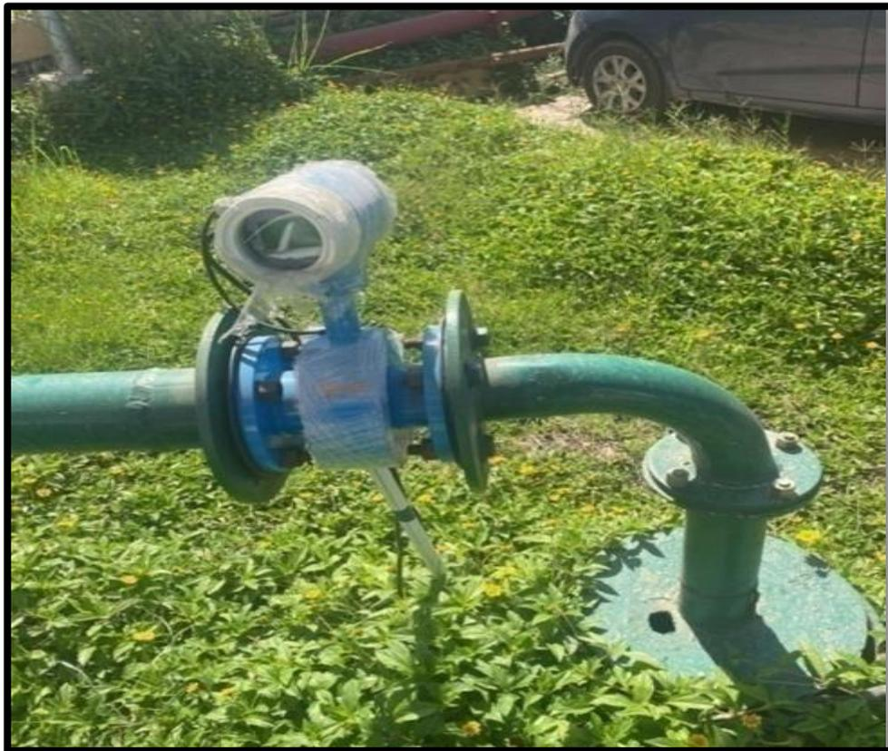
**Tube well installed with electromagnetic flow meter with telemetric module**
