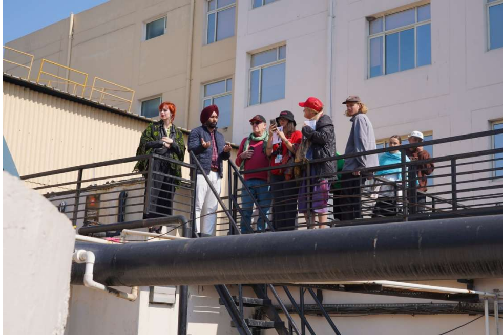
Visit to a Wastewater Treatment Plant, photo captured on 8 th February'24
