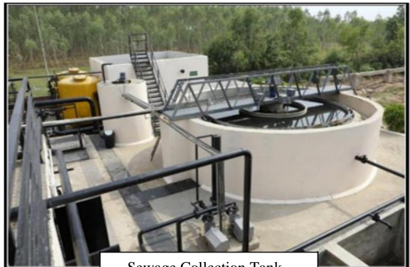
Sewage Collection Tank
